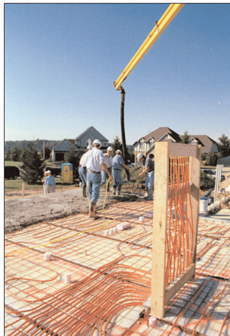
Figure 1. Hydronic radiant floor heating tubing laid out in specific heating pattern prior to concrete pour. Photo courtesy of Ready Mixed Concrete Association of Ontario.
